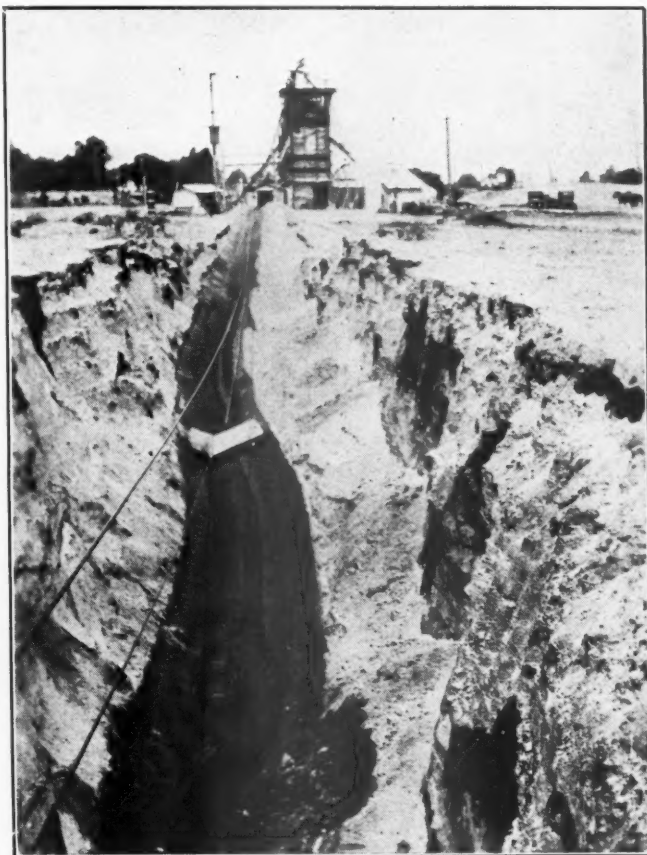
Opening a New Pit at Plant No. 1
